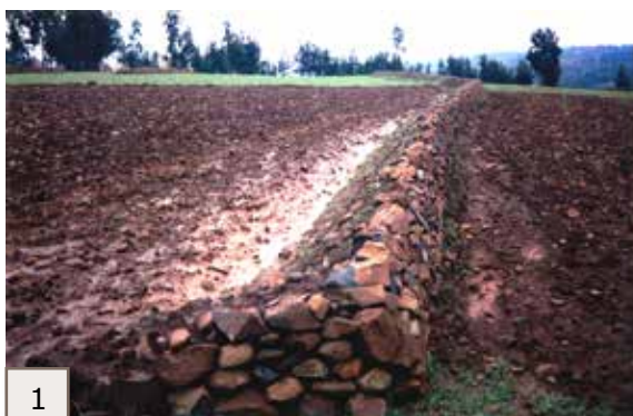
1 Stone faced soil bunds with stable walls
