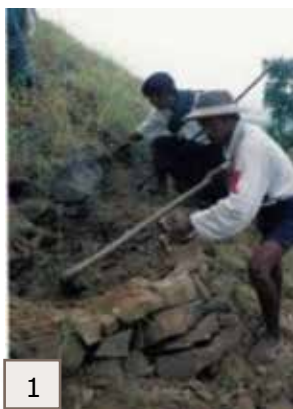
Layout: along contours using A-frame (EB. are built in a staggered position)
