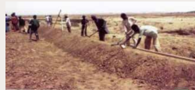
a) Profile of bund and collection trench/ditch - stable soil
