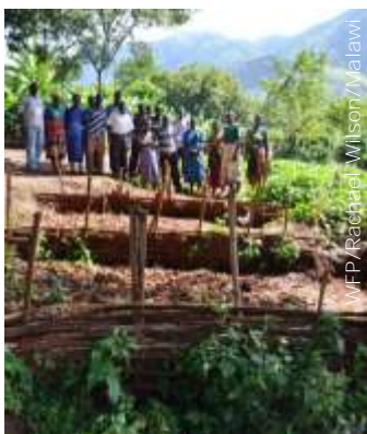
Once a deep gully, the village built these check dams to prevent further erosion along the fields
