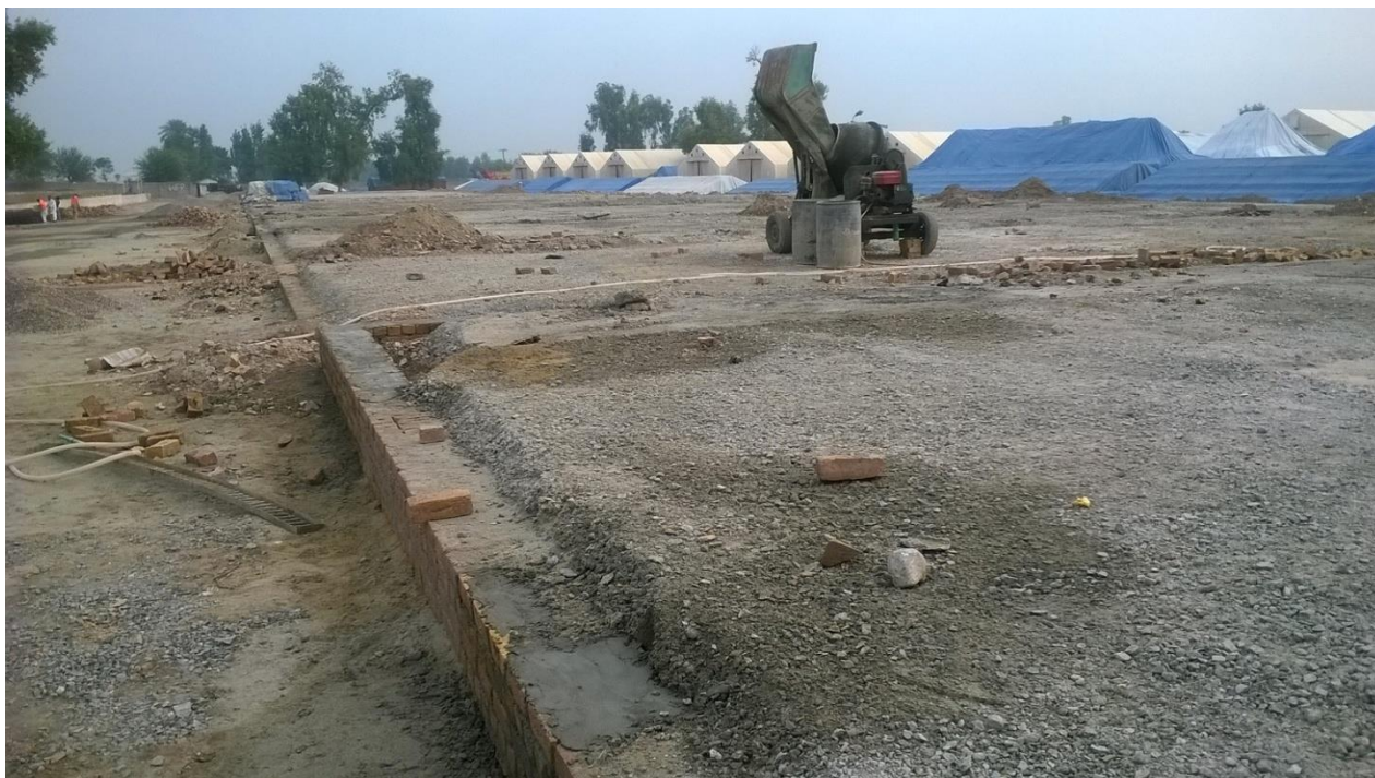
Illustration 3 – Construction of the concrete platform to extend the covered capacity of Nasir Bagh
