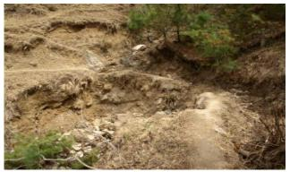
An irrigation channel at Chulakot has several sections where landslips have broken and/or blocked the flow of water. Benefits from this irrigation channel are drastically reduced as a result.
