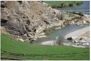
The irrigation channel can be seen along the side of the river. Lack of proper maintenance has left sections in poor condition reducing the benefits to the community.
