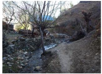
The stone embankment constructed at Dhita is still functioning, but is showing signs of disrepair as there is no active management.
