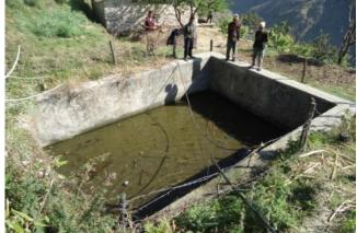
The irrigation pond at Deupatal which is the only pond asset in the VDC to function at all. Most have cracks in the cement and leak.
