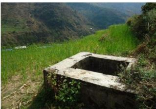
The irrigation water storage tank is an aboveground cement structure and feeds the irrigation system for surrounding land.
