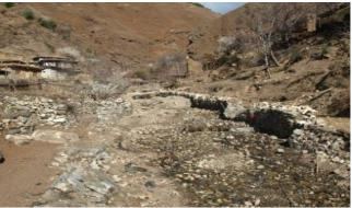
The river embankment strengthening with gabion boxes. This method worked well for some years, reducing the occurrence of flooding. However, lack of maintenance means the threat of flooding has returned as this asset ceases to be functional.
