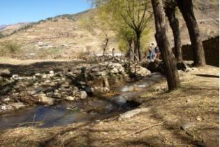
The river embankment is showing signs of dilapidation as maintenance is not carried out. Cattle are believed to cause some damage to the embankment as well as the flood water. Willow trees planted along the river bank are believed to provide a greater bank-stabilising service than the stone embankments built under WFP.
