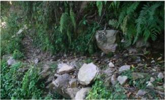
The irrigation channel is incomplete and some places – incomplete sections that are not used are left to fall into disrepair, while completed sections are maintained by their users.
