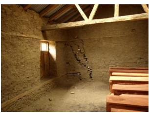
The wall of a school building at Chulakot has a large crack in it. This building is no longer in use by the school for fear of collapse.
