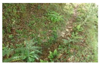
The irrigation channel improved with WFP support provides water for paddy and wheat cultivation. However, as it is earthen and the water source is far away, it is only functional in the rainy season.
