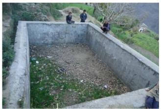
The irrigation pond at Gautarkhal is not functional due to cracks in the cement which causes leakage. No maintenance mechanism is in place to keep the pond in working order. IOD PARC & Rupantaran | VDC Profile | WFP Nepal C/FFA Impact Evaluation
