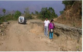
Lack of provision for proper maintenance has left its toll on many sections of road with erosion causing much damage. Here the drainage channel built alongside the road is now above the level of the road it was built to drain water from.
