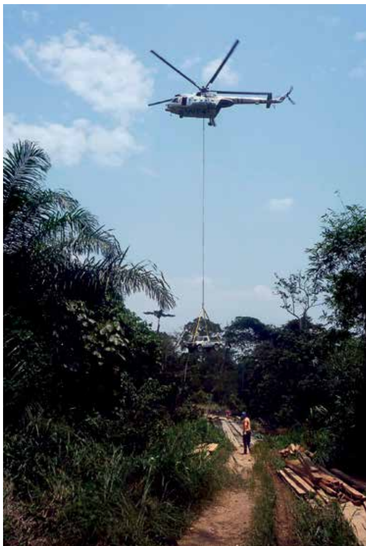
A helicopter sling operation to airlift a stranded vehicle across a bridge for ICRC in DRC, after an accident in 2013
