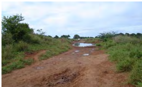
Road damaged by flooding
