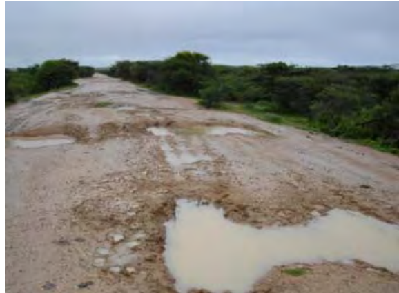
Tarmac and feeder roads are in a poor state
