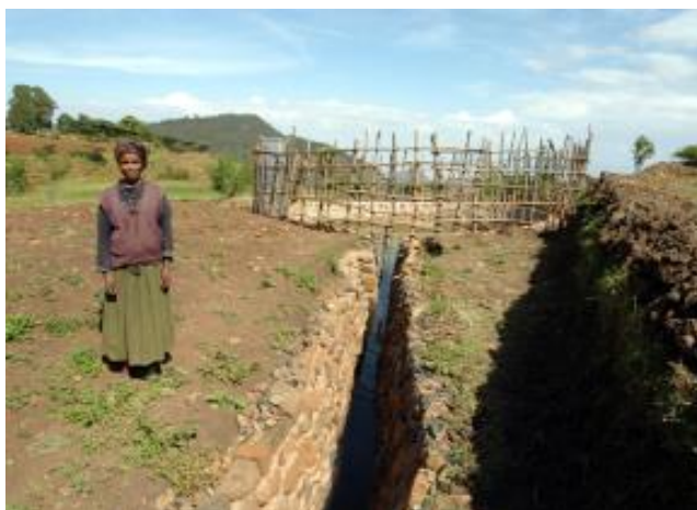
Figure 4.36 - Paved waterway conveying excess runoff into stabilized gullies and water reservoirs (left) and gully control with 'water harvesting check-dams' (right) (Ethiopia – Photos Courtesy by Yonathan Ayalew).
