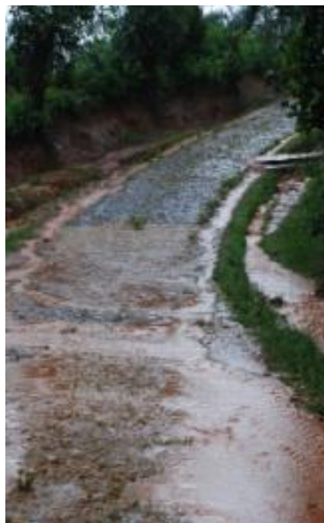
Figure 4.31 - Road temporarily flooded but remaining functional and not damaged (left) (Madagascar, WFP) and feeder road and paved waterway (dual function) in high rainfall and waterlogged prone areas (right) – noticeable is the entry point of the graded stone faced bunds (Ethiopia, MERET -MOA/WFP programme, Photo WFP, V. Carucci).
