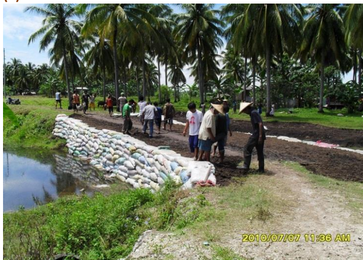
Figure 4.52 - A portion of feeder road-dike strengthened with recycled bags (Philippines, WFP, Photo courtesy by Alemu Mekonnen).
