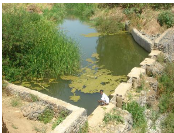
Figure 4.36 - Paved waterway conveying excess runoff into stabilized gullies and water reservoirs (left) and gully control with 'water harvesting check-dams' (right) (Ethiopia – Photos Courtesy by Yonathan Ayalew).
