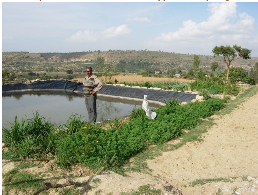
Figure 4.17 - Micro-ponds constructed around homesteads (lined with plastic geo-membranes) collect runoff water from micro-catchments (from road sides, grassed or rocky areas) that can be used for horticulture after the rainy season or to supplement additional water to vegetable and cash crops during and after the main rainy season (Eastern Tigray, Ethiopia, MOA-WFP, MERET programme, Photo WFP, V. Carucci).
