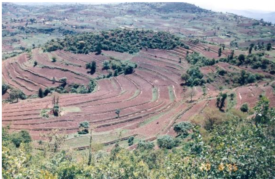
Figure 4.16 - Soil bunds precisely constructed along contour lines - water collected above the bunds can be noted – this creates a percolation effect that moisturizes the entire area, particularly the first few meters above the terrace (W.Hararghe zone, Ethiopia, MOA-WFP, MERET programme, Photo courtesy Lakew Desta).
