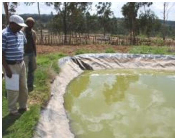
Figure 4.35 - Micro-ponds (left) (small sized micro-pond for individual users, approx. 60 m 3 ), and large micro-pond for group of households , approx. 500 m 3 (right) (Ethiopia, MERET – MOA/WFP, Photo WFP, V. Carucci).
