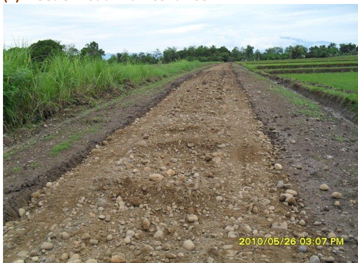
Figure 4.53 - Side drains dug and filled for better designed camber shaped road (Philippines, WFP – Photo courtesy by Alemu Mekonnen).
