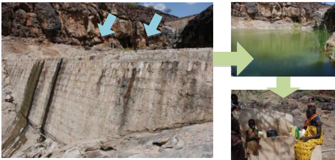
Figure 4.8 - Rock catchment water scheme - a cemented dam collecting water in depression points (WFP-World Vision, Turkana, Kenya). A water collection system with pipes and taps is established downstream. (Photo WFP, V. Carucci).
