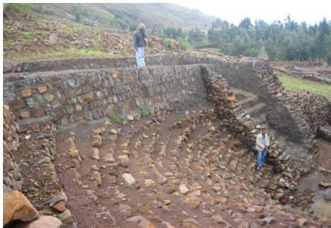
Figure 4.62 - SSD with reinforced spillway and drop structures in V-shaped gullies (Ethiopia, Amhara region–MERET, MOA/WFP - Photos Courtesy by Yonathan Ayalew).
