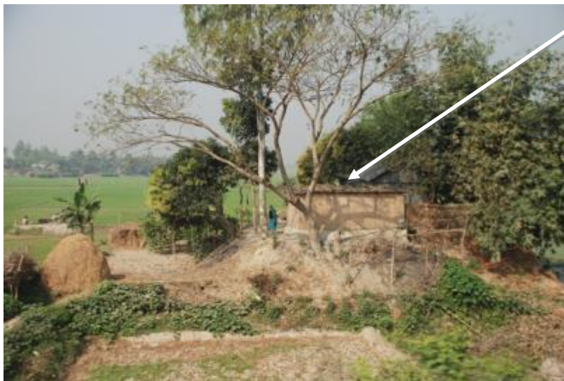
Figure 4.46 - Raised ground with a homestead on top – this activity is not done on isolation but integrated within larger flood protection measures, often on top of existing raised grounds and embankments (Bangladesh, Photo V. Carucci).
