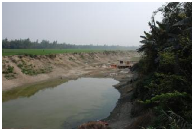
Figure 4.44 - Main excavation on drainage lines for protection against seasonal flooding of homesteads and of rice fields (Source WFP).
