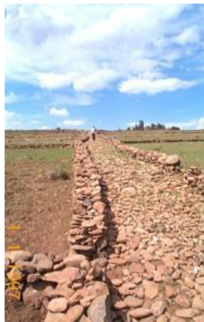
Figure 4.31 - Road temporarily flooded but remaining functional and not damaged (left) (Madagascar, WFP) and feeder road and paved waterway (dual function) in high rainfall and waterlogged prone areas (right) – noticeable is the entry point of the graded stone faced bunds (Ethiopia, MERET -MOA/WFP programme, Photo WFP, V. Carucci).
