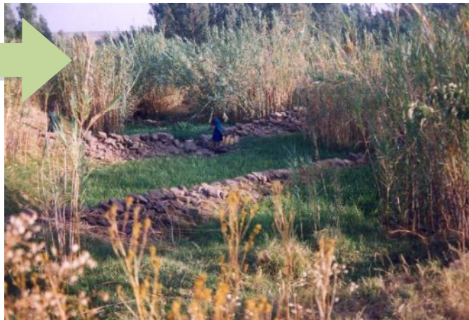
Figure 4.63 – Head of gully with stepped stone riser and checkdams and grasses (MERET, MOA/WFP, Photos WFP, V. Carucci).
