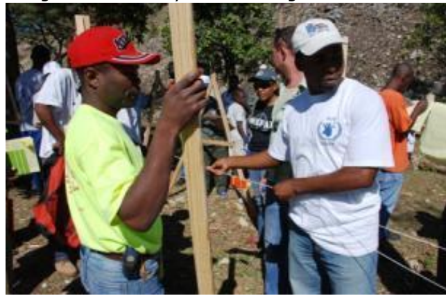
Using line level for layout of soil bunds
