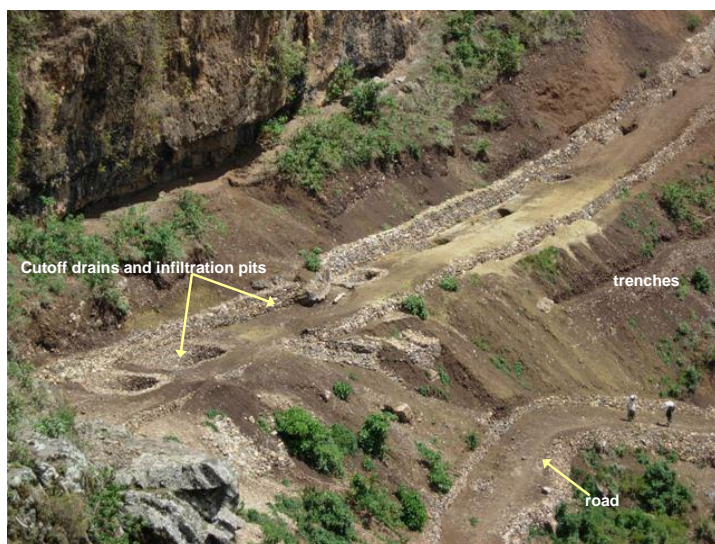
Figure 4.30 - Road protection systems – side drains and runoff control systems for major tree planting and stabilization built above the constructed road in high rainfall areas (high/medium altitude) – (MERET, Amhara region of Ethiopia, MOA/WFP, Photo WFP, V. Carucci).
