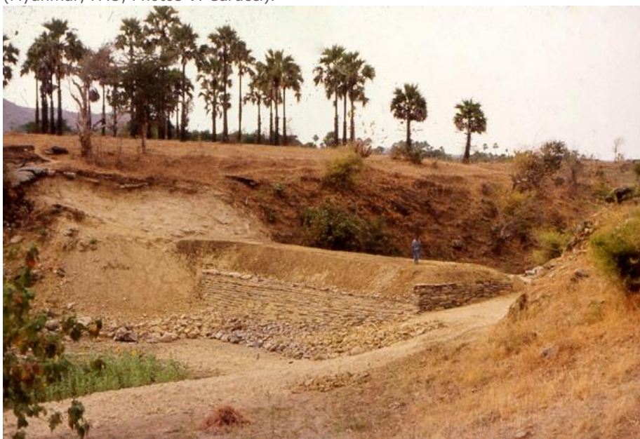
Figure 4.64 - Upstream side of SSD in large gullies (Myanmar, FAO, Photos V. Carucci).
