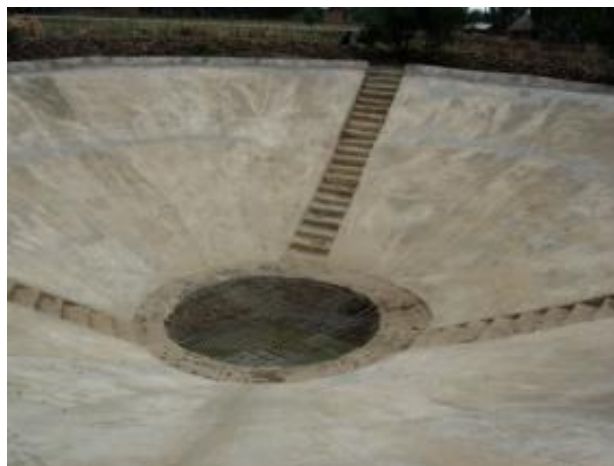
Figure 4.36 - Paved waterway conveying excess runoff into stabilized gullies and water reservoirs (left) and gully control with 'water harvesting check-dams' (right) (Ethiopia – Photos Courtesy by Yonathan Ayalew).
