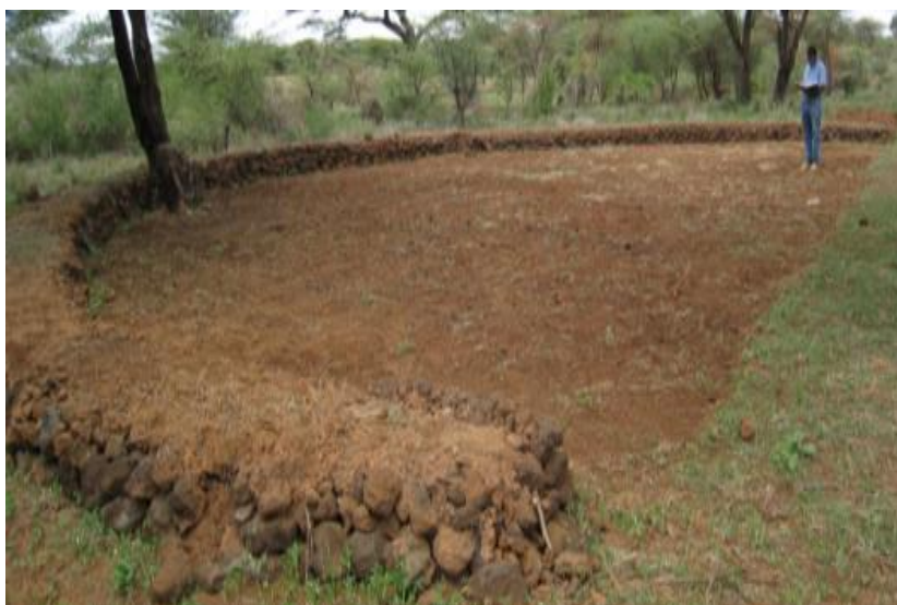
Figure 4.19 - Semi-circular bund constructed in Chumvi Yare, Isiolo district of Kenya, WFP, Photo B. Tefera).
