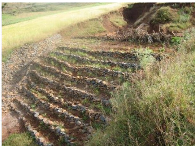
Figure 4.61 - Stone stepped & soil filled SSD planted with grasses and with stone paved spillway.
