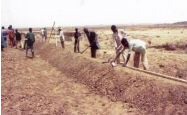
Checking top level of soil bund using A-frame
