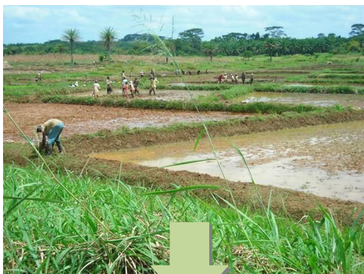
Figure 4.42 - Formerly abandoned irrigation schemes cleared from overgrown vegetation, with irrigation canals re-lined up and bunds reconstructed (Liberia, Livelihood Asset Rehabilitation programme - LAR, photos WFP, V. Carucci).
