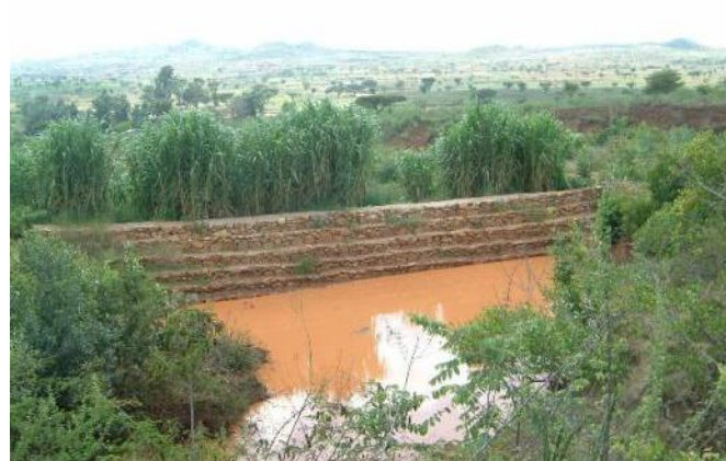
Figure 4.60 - A soil sedimentation and overflow dam filled up with soil and planted with forage shrubs (Ethiopia, SNNPR region – MERET, MOA/WFP - Photo WFP, V. Carucci).
