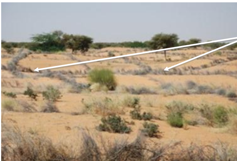
Figure 4.24 - Sand dunes stabilized with dry fences/grids and recently planted with trees (WFP-MOE, Diffa region – Niger, Photo WFP, V. Carucci, WFP).
