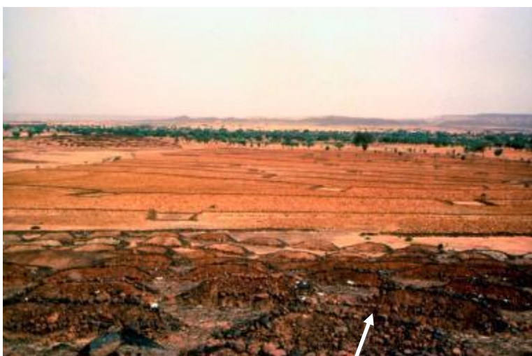
Figure 4.6 - Trenches and stone faced bunds in dry and bare sub-watersheds.
