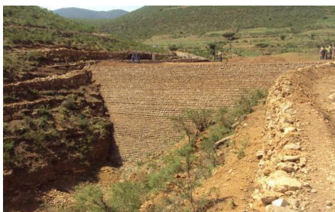
Figure 4.59 - Soil Sedimentation and overflow dam across a large gully using dry masonry (Ethiopia, Dire Dawa region – MERET, MOA/WFP, Photo WFP, V. Carucci).
