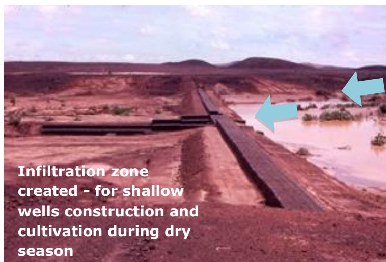
Figure 4.7 - A gabion and soil (laterite) percolation dam constructed across large river beds/drainage lines.
