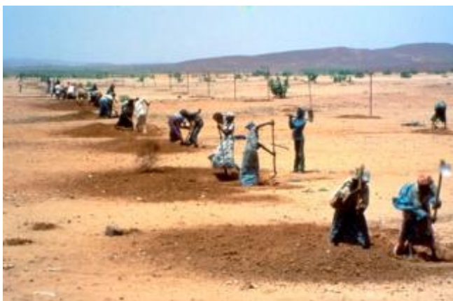
Figure 4.3 - Semi-circular basins for reforestation in Niger (Keita Project – FAO/ITA with WFP support for FFW activities in the 1990's, Photo source - FAO)
