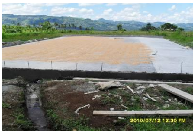
Figure 4.57 - A solar drier, including cemented floor and side drains
