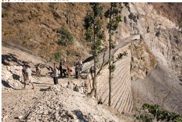
Figure 4.54 - Road construction in steep mountainous terrains – strong walling and reinforcements applied (Nepal, source WFP).
