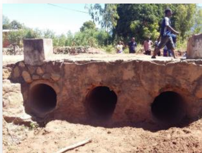
A road rehabilitated by relief beneficiaries
